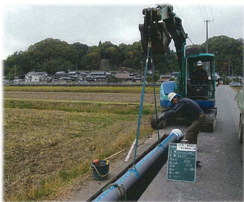
◆耐震管の布設◆
