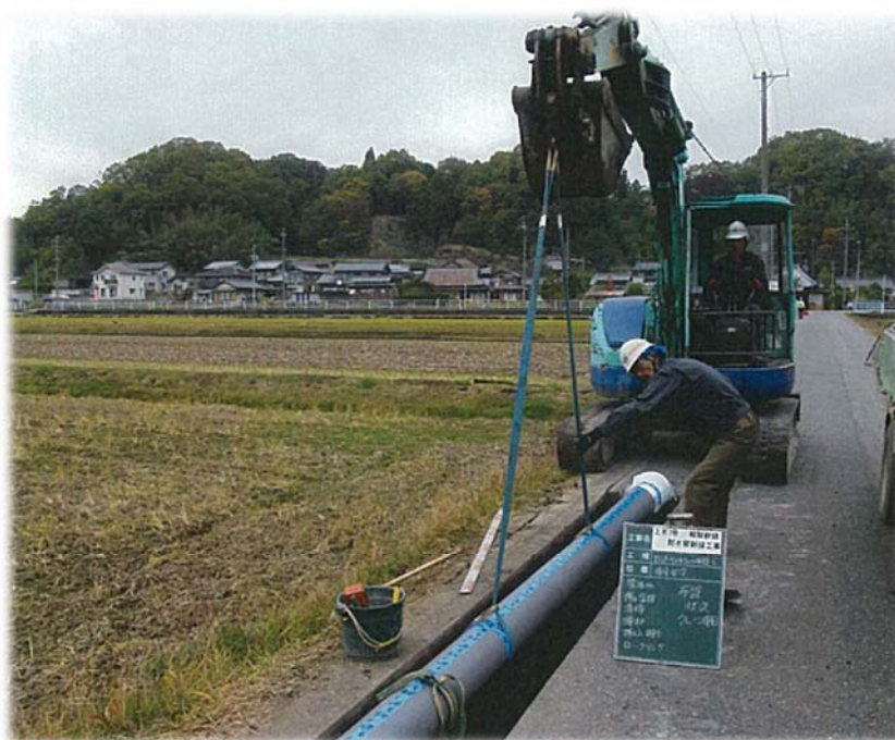
◆耐震管の布設◆
